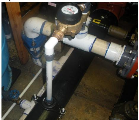
A system water meter was installed between the pressurized line and the distribution system. This low-volume meter is rated at 25 gallons/minute. With 2 valve changes, all water used in the system is routed through this meter. By isolating varous sectors and comparing flow rates, excess water use can be located by sector.
