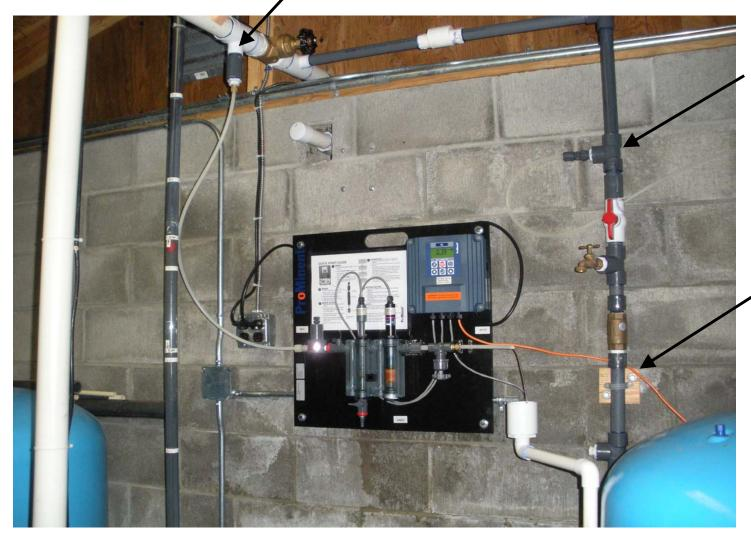
WELL CYCLE CHLORINE INJECTION POINT - BRINGS INCOMING WELL WATER TO 0.34 PPM CHLORINE
