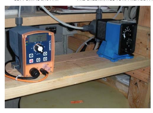
THESE INJECTION PUMPS COMBINE TO PROVIDE 0.40 PPM (0.20 - 2.00 PPM REQUIRED)
