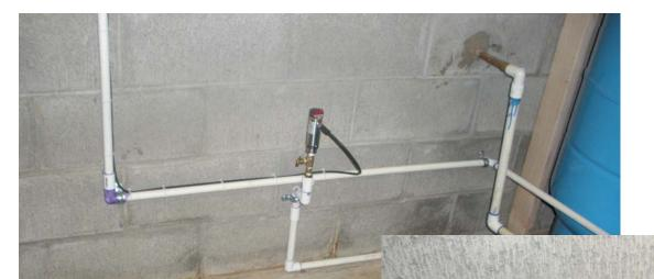
A TRANSDUCER PRESSURE UNIT IS NOW USED TO CONTROL THE WELL CIRCUIT, PREVIOUSLY DONE WITH A FLOAT SWITCH IN THE RESERVOIR.
