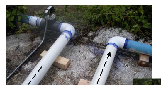
THE FLOW FROM THE WELLS TO THE RESERVOIR IS DIVERTED THROUGH THE MIXING MANIFOLD, WHERE THE POLYPHOSPHATE IS INJECTED AND MIXED. THE MIXING OCCURS PRIOR TO THE WELL WATER ENTERING THE RESERVOIR. THE CLORINE INJECTION TAKES PLACE AT THE RESERVOIR INLET.
