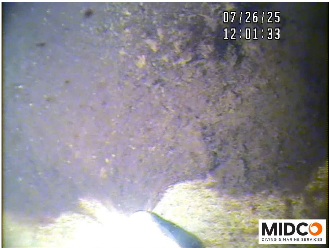
Cleaning Reservoir – Up to 10" of Sediment Noted
