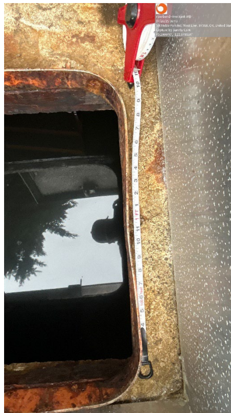
Access Hatch – Corrosion Noted
