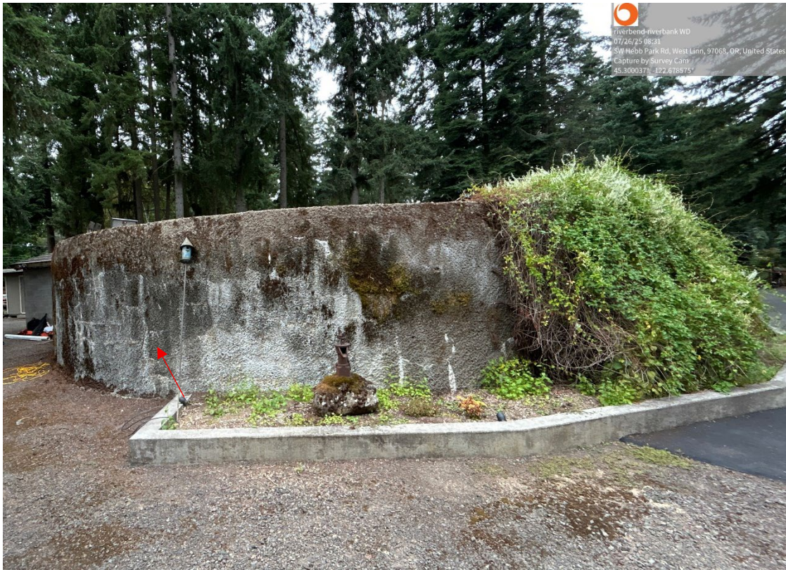
Exterior Reservoir – Settling Cracks & Biological Growth Noted
