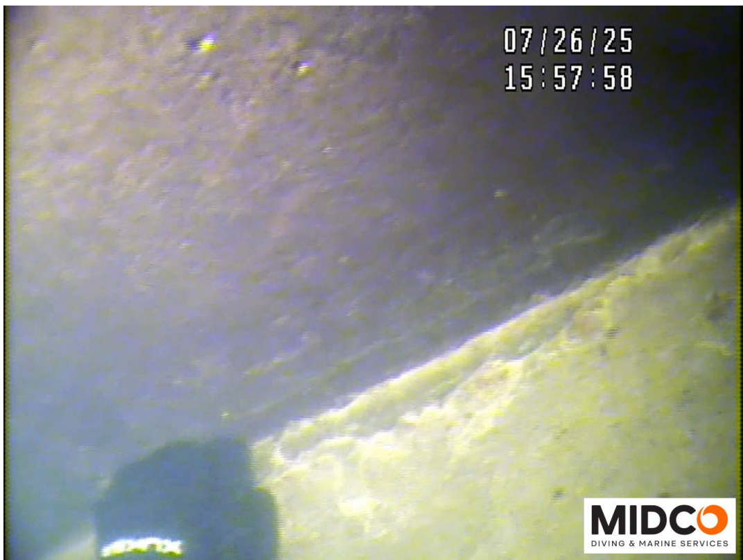
Floor to Wall Seam – Settling Cracks & Spalling Noted
