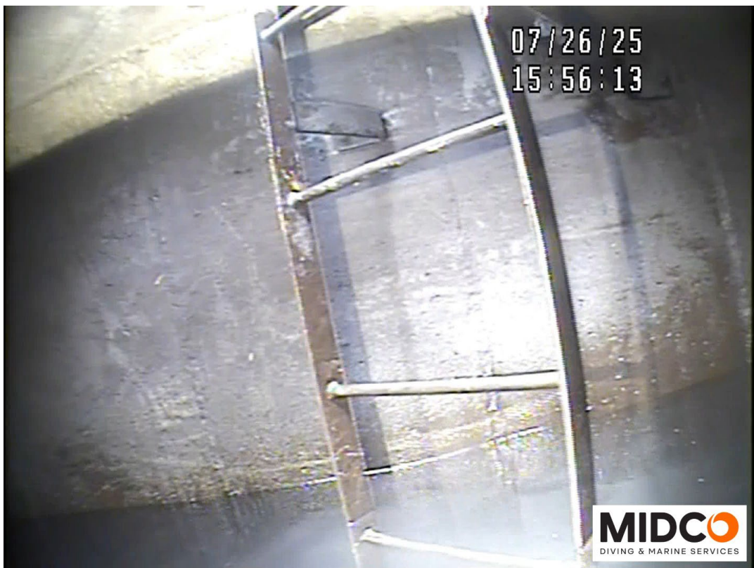
Interior Ladder – Corrosion Noted
