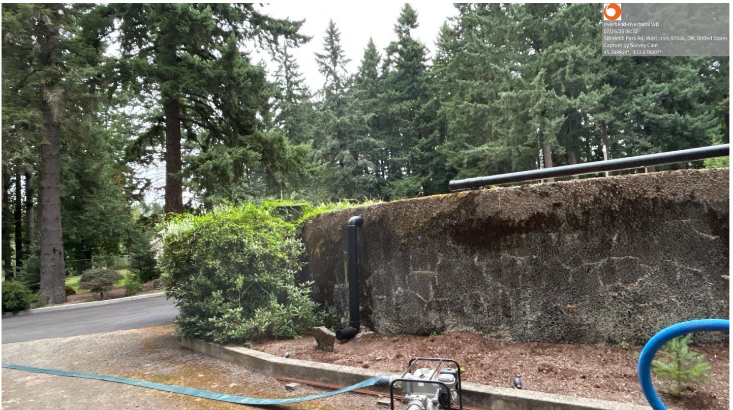
Exterior Reservoir – Settling Cracks Noted
