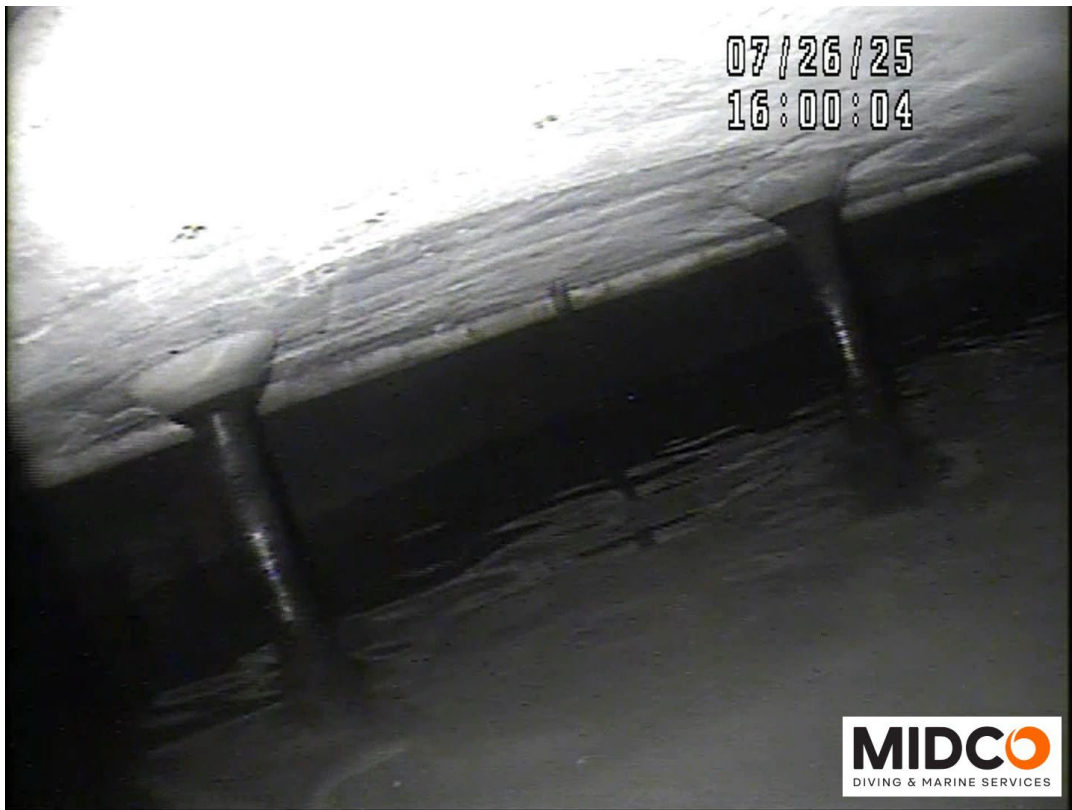
Typical Roof – Exposed Rebar with Corrosion Noted
