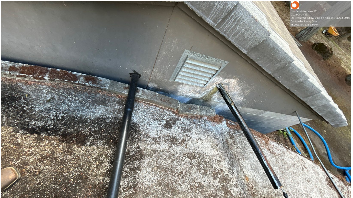
Exterior Roof – Evidence of Water Migration Noted
