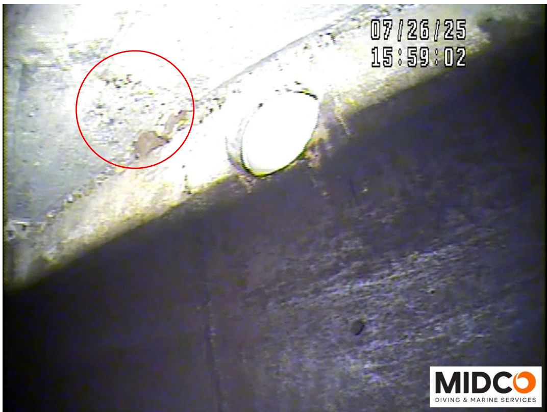
Overflow Plumbing & Wall to Roof Seam – Spalling Noted
