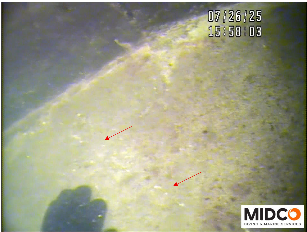
Typical Floor – Settling Cracks with Efflorescence Noted
