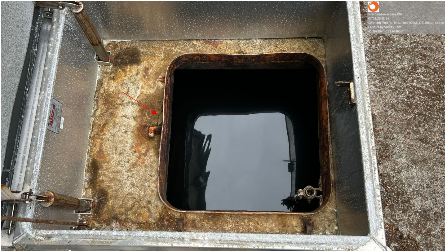
Access Hatch – Settling Cracks & Corrosion Noted
