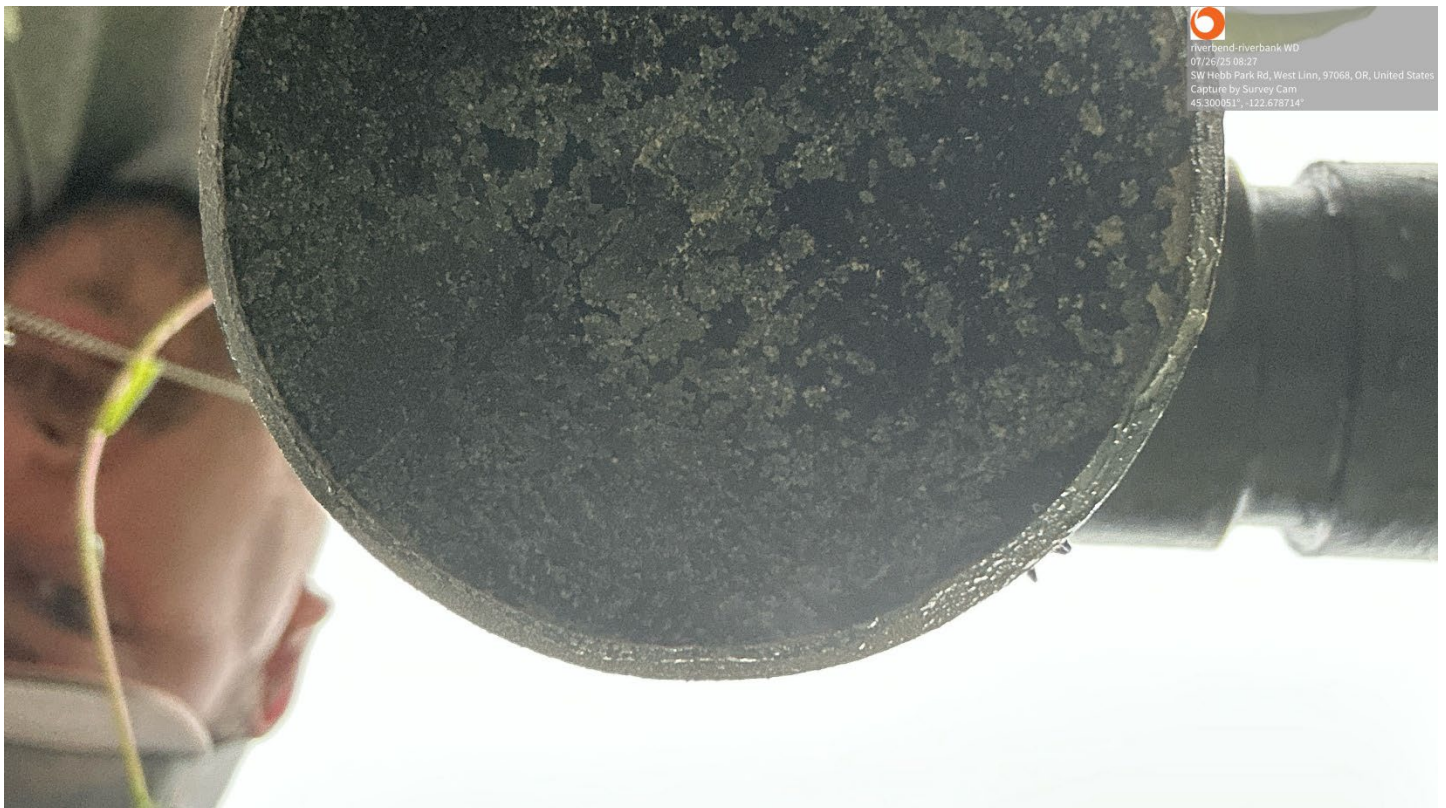
Roof Vent Screen – Blockage Noted
