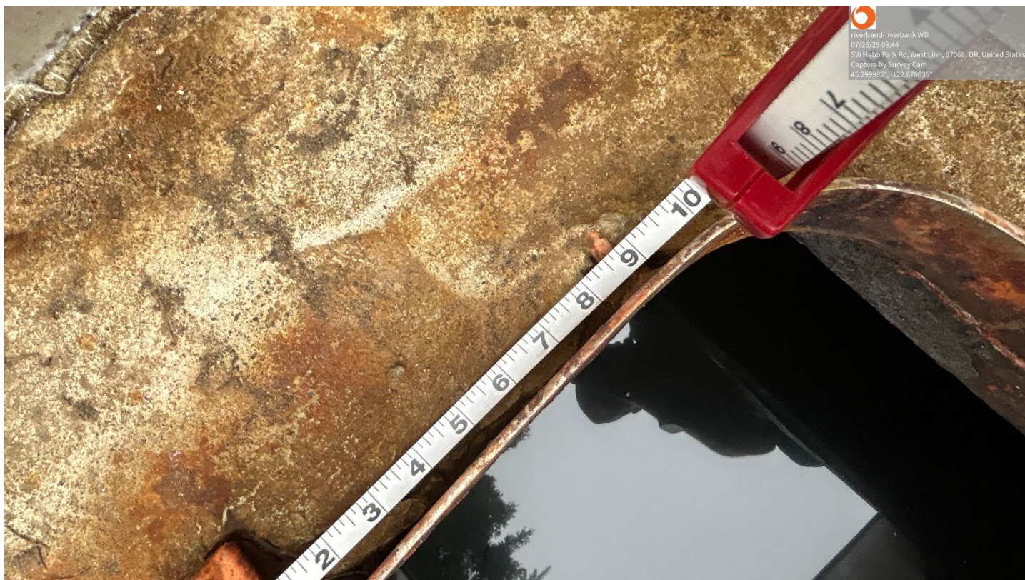
Access Hatch – Corrosion Noted
