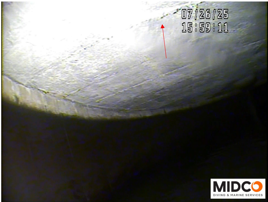
Wall to Roof Seam – Settling Cracks & Spalling Noted
