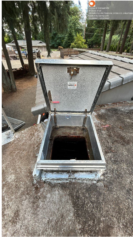
Access Hatch – Weather Stripping Deterioration Noted
