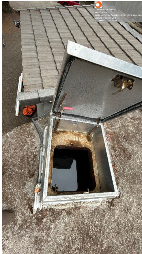
Access Hatch – Corrosion Noted
