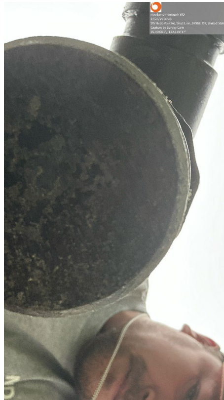
Roof Vent Screen – Biological Growth Noted
