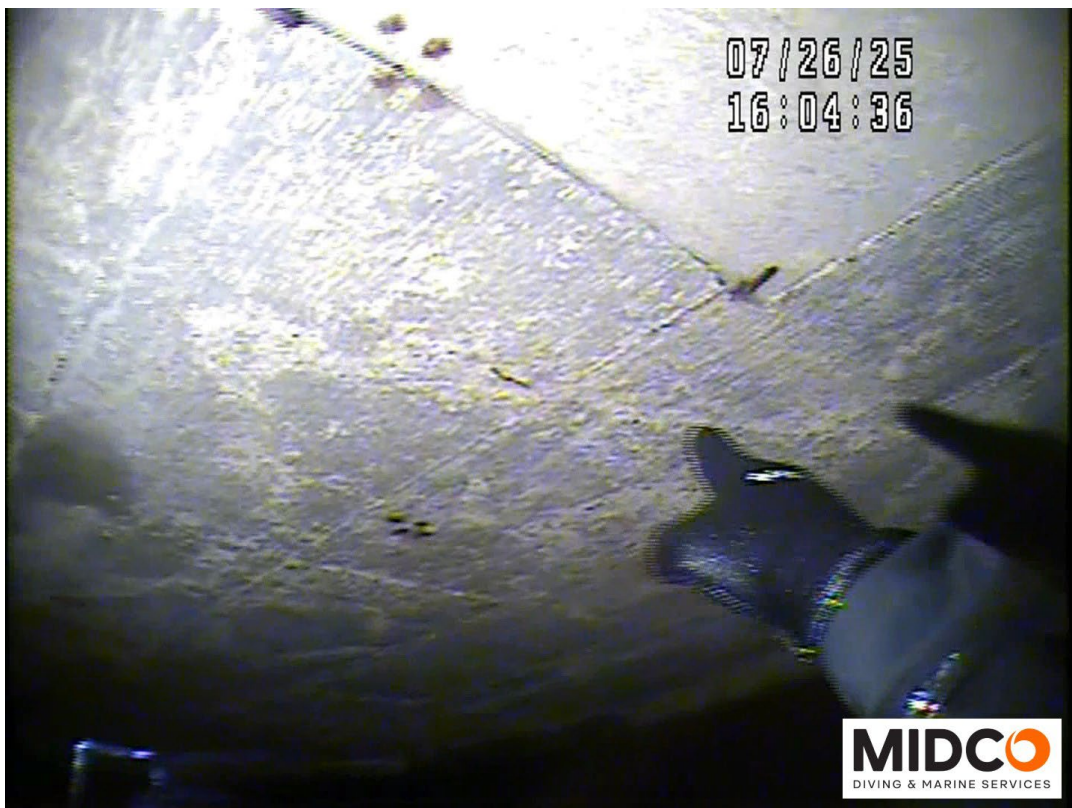
Typical Roof – Exposed Rebar with Corrosion Noted
