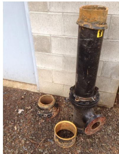
PART OF THE IRON PIPES REMOVED
