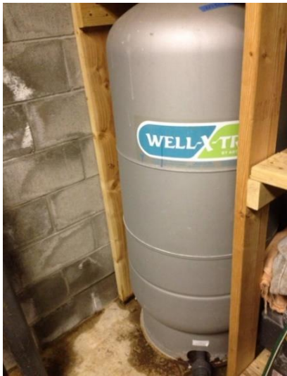
OLD PRESSURE TANK REMOVED
